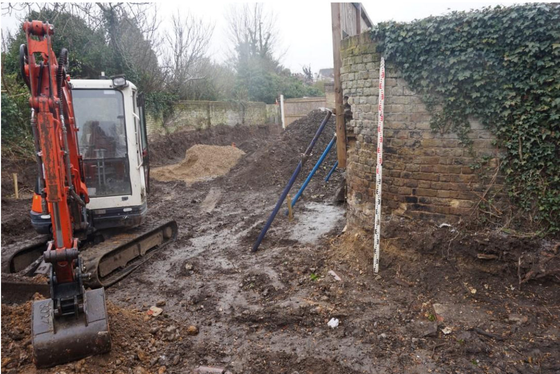
Plate 2: Looking south at the site from north end
