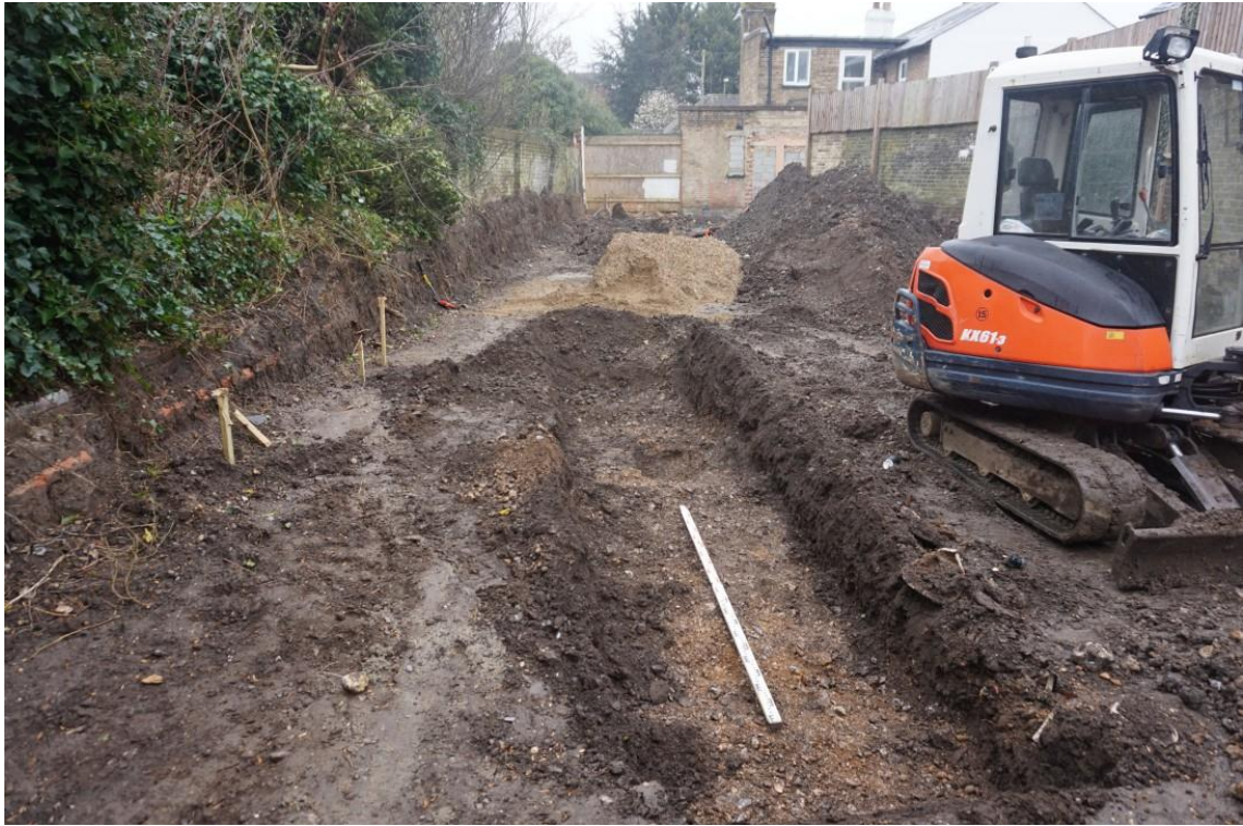
Plate 5: Looking south at Trench 2
