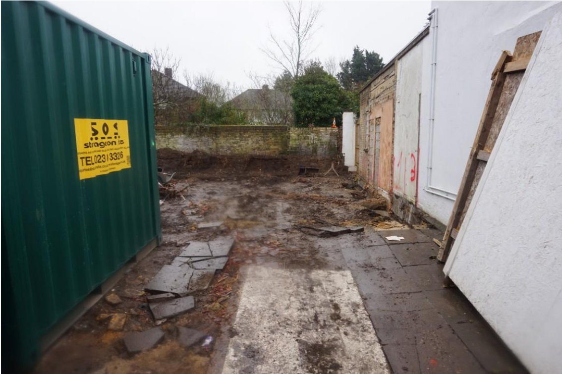
Plate 1: Looking east at the south side of the site. Paint on the wall to the right indicate location of recently demolished building
